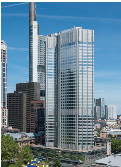
SSM (Single Supervision Mechanism), Eurotower, Frankfurt
